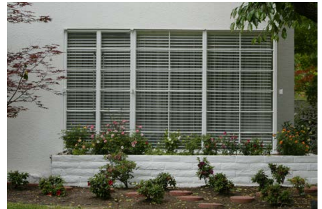
Casement Windows. If ever replaced, the pattern, size and shape of these casement style windows should be maintained.
