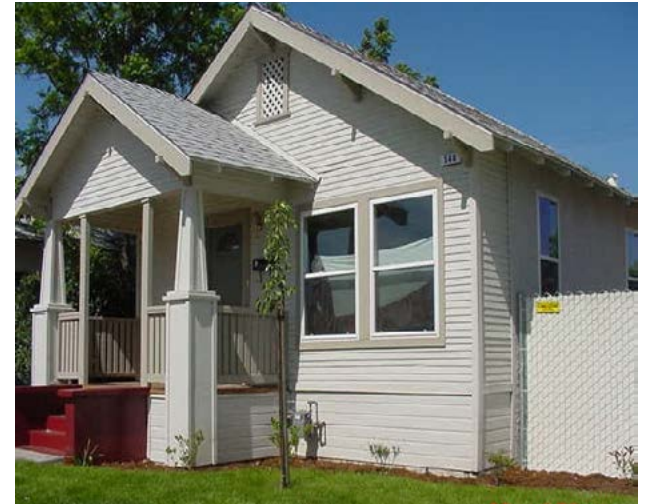
Renovated Façade on Palm Avenue Bungalow.
