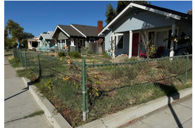
Chain Link Fencing. Chain link fencing is prohibited as front yard fencing in the Tower District.
