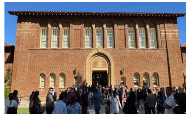
The Administration Building at Fresno Community College offers an excellent example of the Renaissance Revival architectural style, which is characterized by symmetrical rhythms, grand entrance, and small windows on the ground floor.
