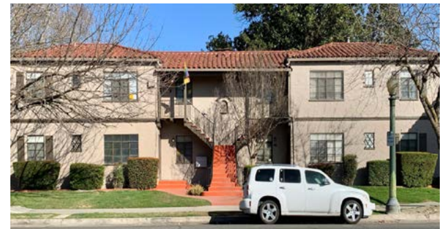
Early 20th-century apartment building with covered entry and varied massing.
